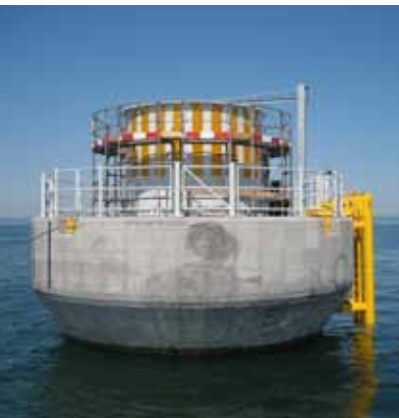
Lillgrund Offshore Wind farm, Sweden
