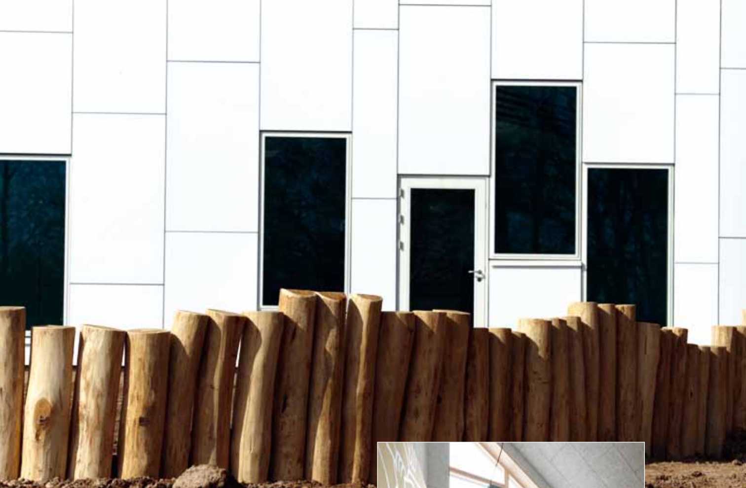
Designbørnehaven "Paletten", Kolding / Kindergarden "Paletten", Kolding, Jutland
