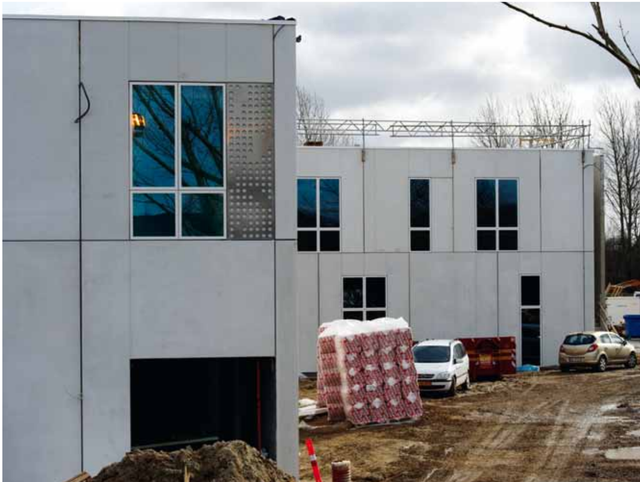
Tornbjerg Gymnasium, Odense / Tornbjerg Upper Secondary School, Odense
